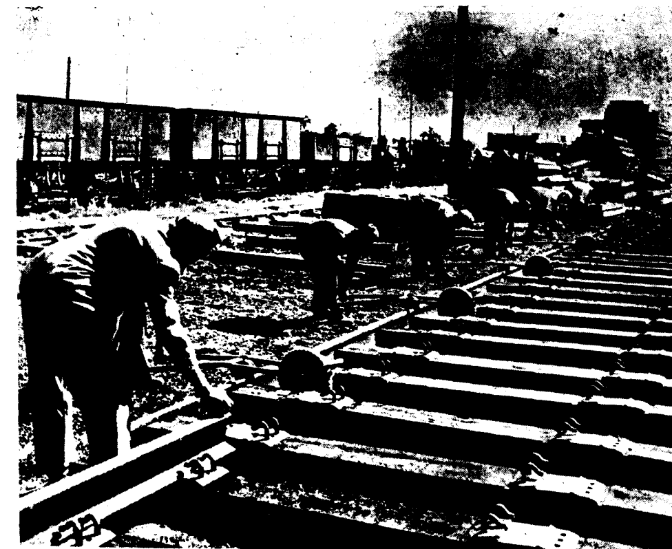
Rail on ground at sleeper ends.
