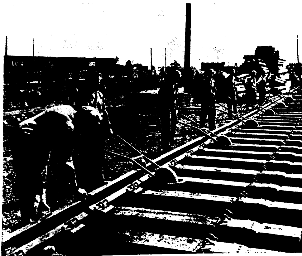
Rail into chairs, or on to base-plates.
