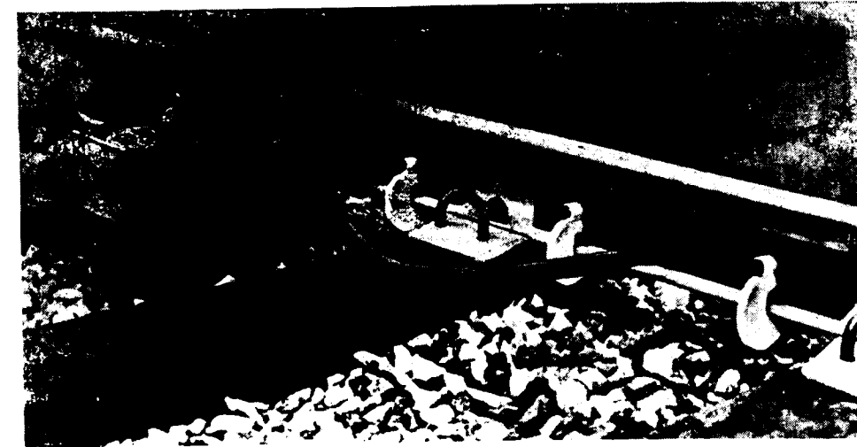
"Mills Hurcol" Lubricator Mounted Inside the Track.
