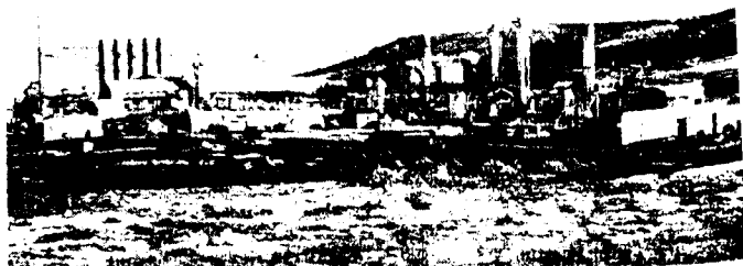
13. Sulphur from natural gas: from a daily output of 60 million cubic feet of natural gas at Jumping Pound, Alberta, 80 tons a day of sulphur are extracted.
