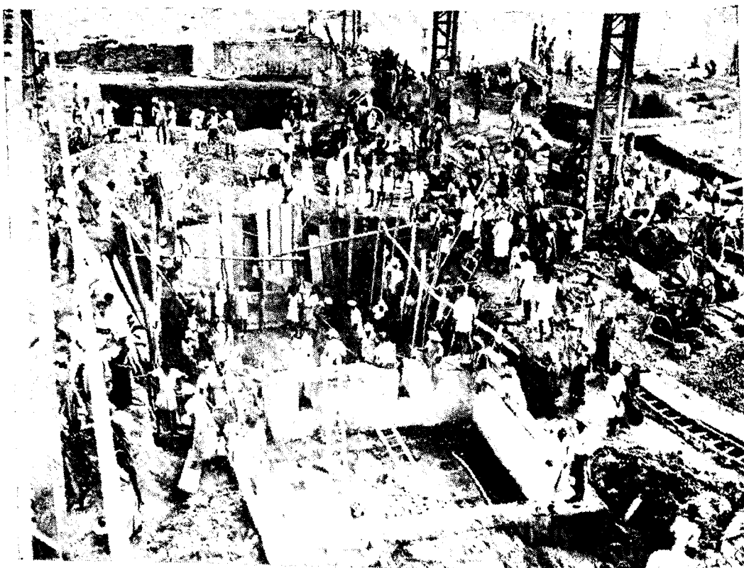
Heavy foundations for the Beche Smithy Hammers being done under difficult subsoil conditions. The foundations rest on groups of 25 piles
