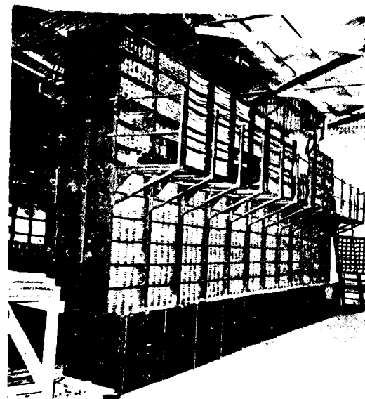
A view of the Main Stores Depot showing 15 ft. high Steel Racks
