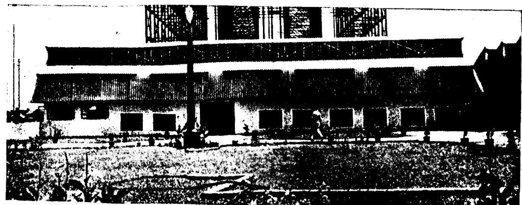
Exterior view of the Technical Training School of the Integral Coach Factory, Perambur
