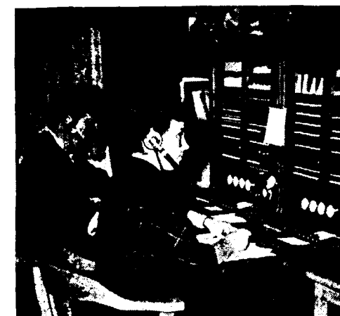
The busy telephone exchange of the European central wagon control at Berne, Switzerland
