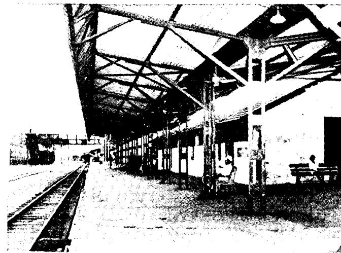
Roofing over the Island Platform at Renigunta Jn.
