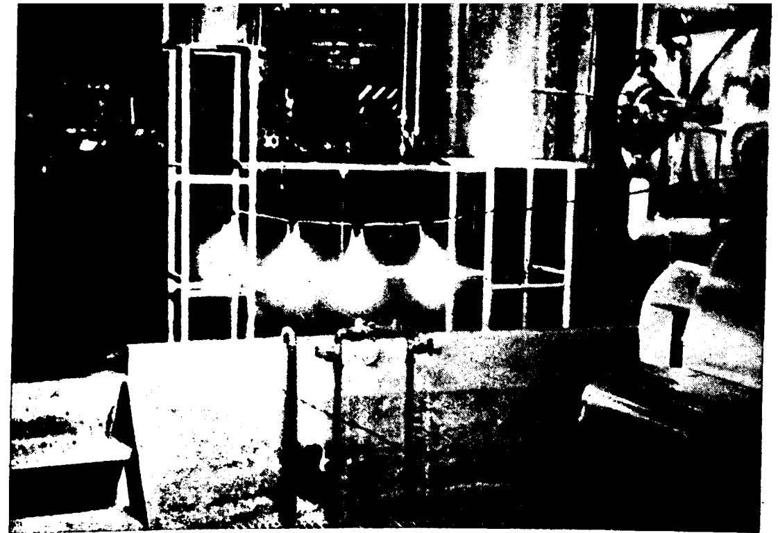
The electric light bulbs here show the first known use of electric power from atomic energy. The generator is run by a turbine which uses steam produced by means of heat supplied by the Experimental Breeder Reactor located at Idaho Falls in the United States
