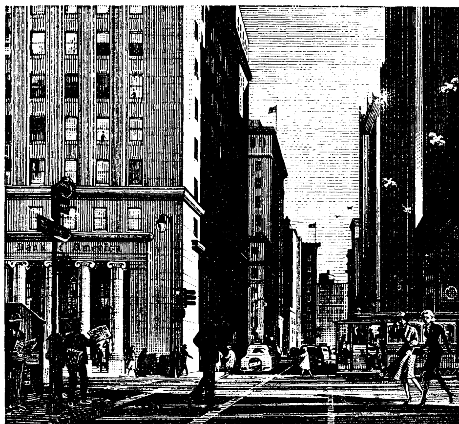
Bank of America Head Office San Francisco, California
