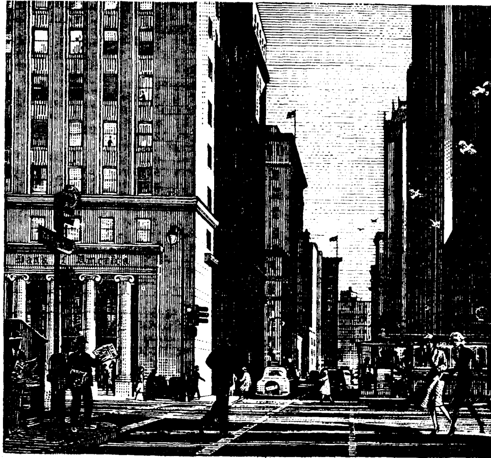
Bank of America Head Office San Francisco, California
