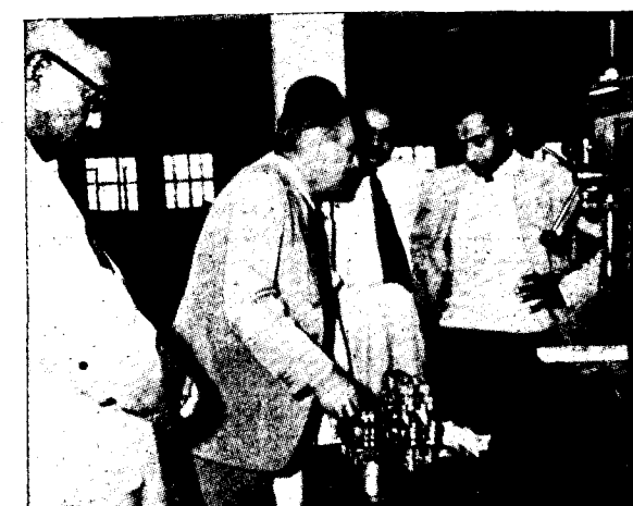
Mr. P. C. Mukherjee, Member Engineering Railway Board, inspecting contactor switches in the process of manufacture.
