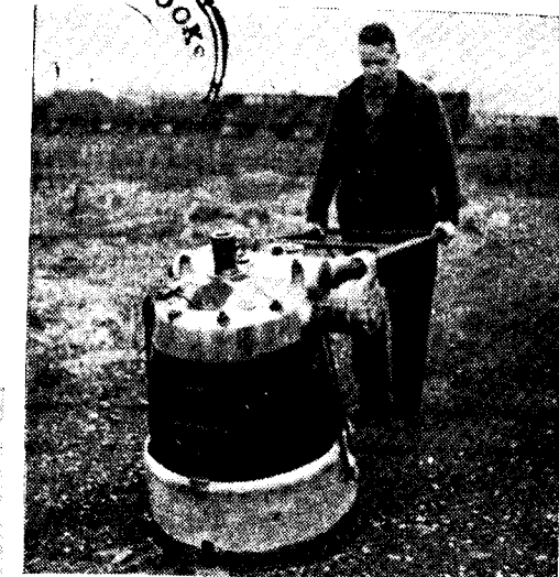
Big Problems — The Johnson Frog Rammer is suitable for Earth Dams, Bunds, Canal Work, Railway Embankment, etc.
