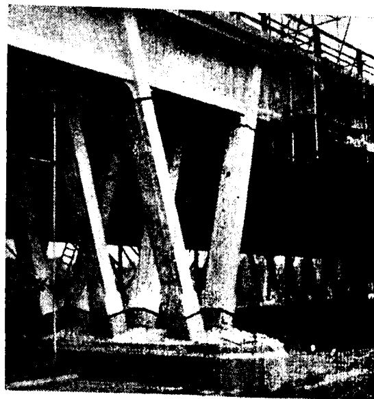
The bridge over the River Dendre, near Alost. (Belgium) The lower photograph shows the V-shaped supports, formed of inclined struts hinged top and bottom.
