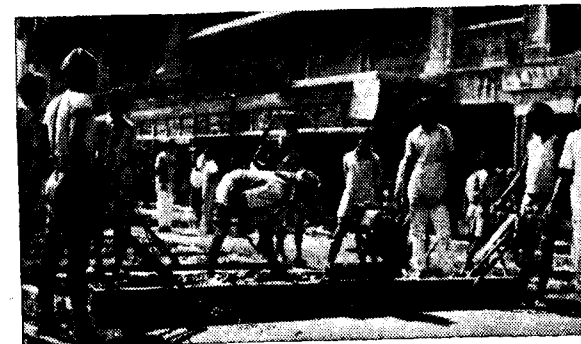
C. H. Johnson self-propelled screed vibrator.
