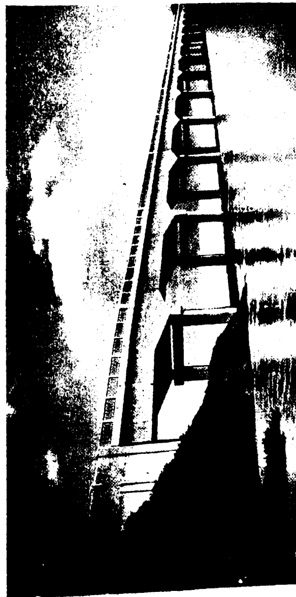
KIUL BRIDGE —Recently designed and constructed over the Kiul River on the Patna Ranchi Indian National Highway near Jamul. The bridge has a total length of 1,198 ft. 6 ins. with a cantilever type R.C.C. beam and slab superstructure carrying a 22 ft. clear roadway and resting on R.C.C. piers spaced 89 ft. and 87 ft. 9 ins. apart. The bridge foundations consist of two 14 ft. diameter masonry wells under each pier, sunk down by open grabbing up to 60 feet below bed level.
