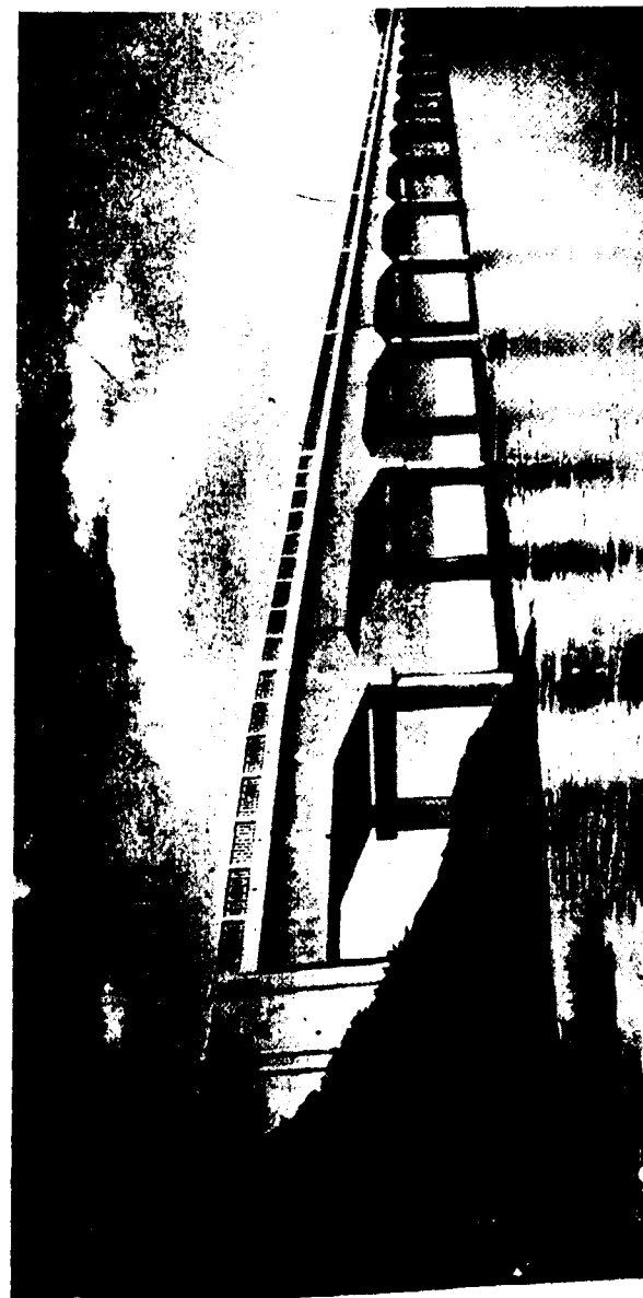
KIUL BRIDGE —Recently designed and constructed over the Kiul River on the Patna Ranchi Indian National Highway near Jamui. The bridge has a total length of 1,198 ft. 6 ins. with a cantilever type R.C.C. beam and slab superstructure carrying a 22 ft. clear roadway and resting on R.C.C. piers spaced 89 ft. and 87 ft. 9 ins. apart. The bridge foundations consist of two 14 ft. diameter masonry wells under each pier, sunk down by open grabbing up to 60 feet below bed level.
