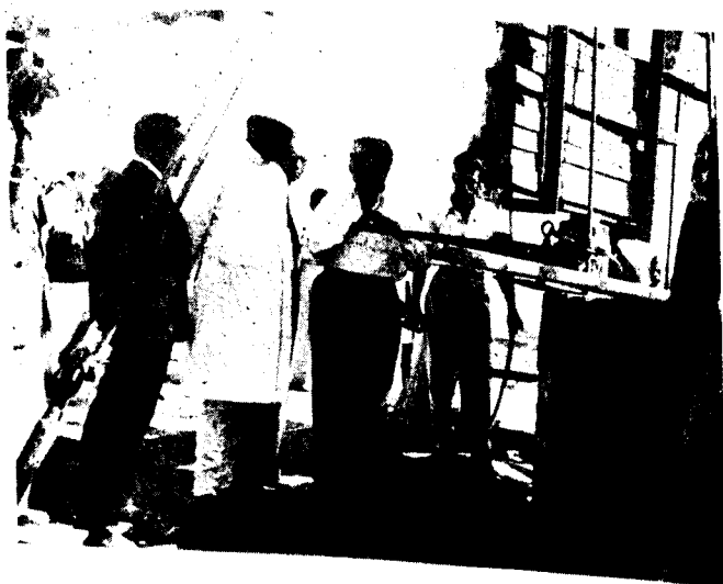
Photo 5: Dr. Jivraj Mehta—Minister for P.W.D. Bombay inspecting the Jack arrangement.
