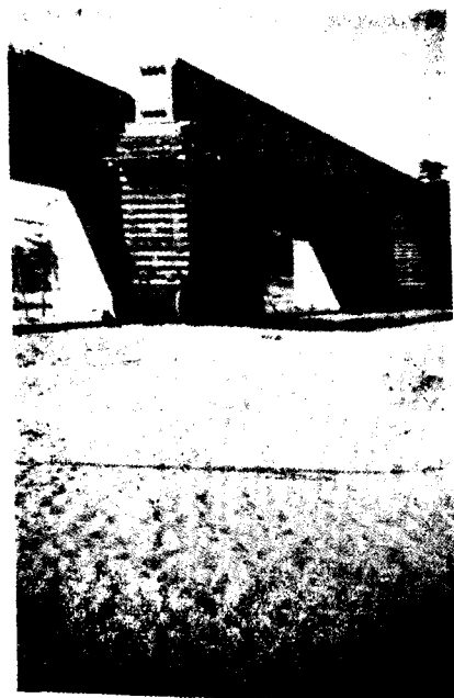
Photo 19. A beam on the move on the river bed
