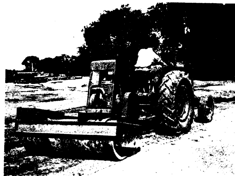
Photo 2. Vibrating Roller at work
