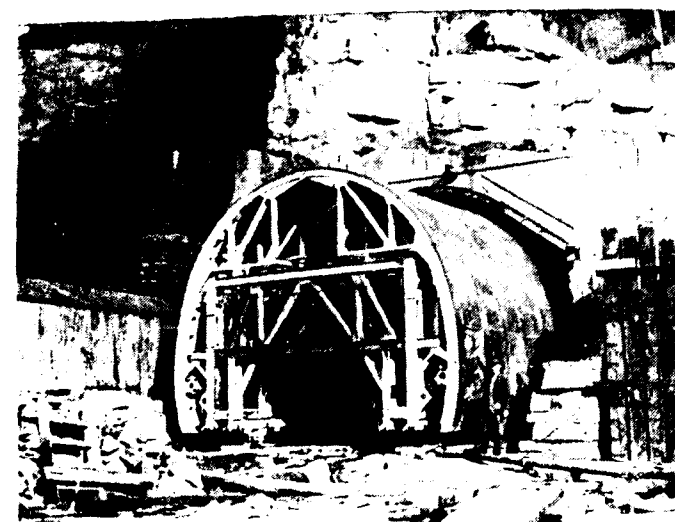
First 20-foot section of travelling steel shutter assembled at Woodhead.
