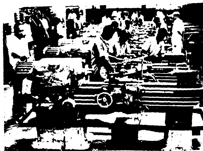
Batch of RL lathes under erection.
