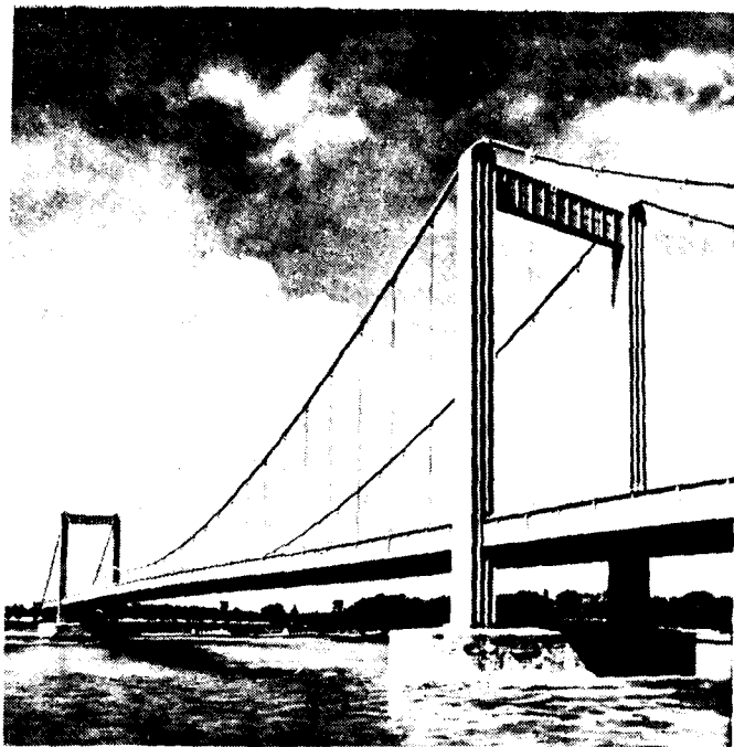
Super-Highway Bridge Cologne-Rodenkirchen, span 310 ft. 1 in. + 1240 ft. 2 in + 310 ft. 1 in. steel weight 12,300 l. ts.
