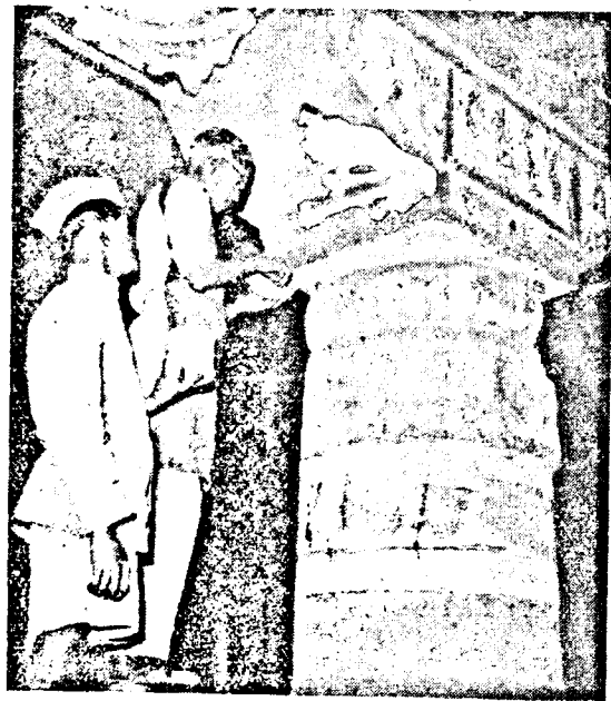
Conservation staff of the Archaeological Department of the Government of India removing the dust, after scraping the edges of the damaged portion of the frescoes at Ajanta
