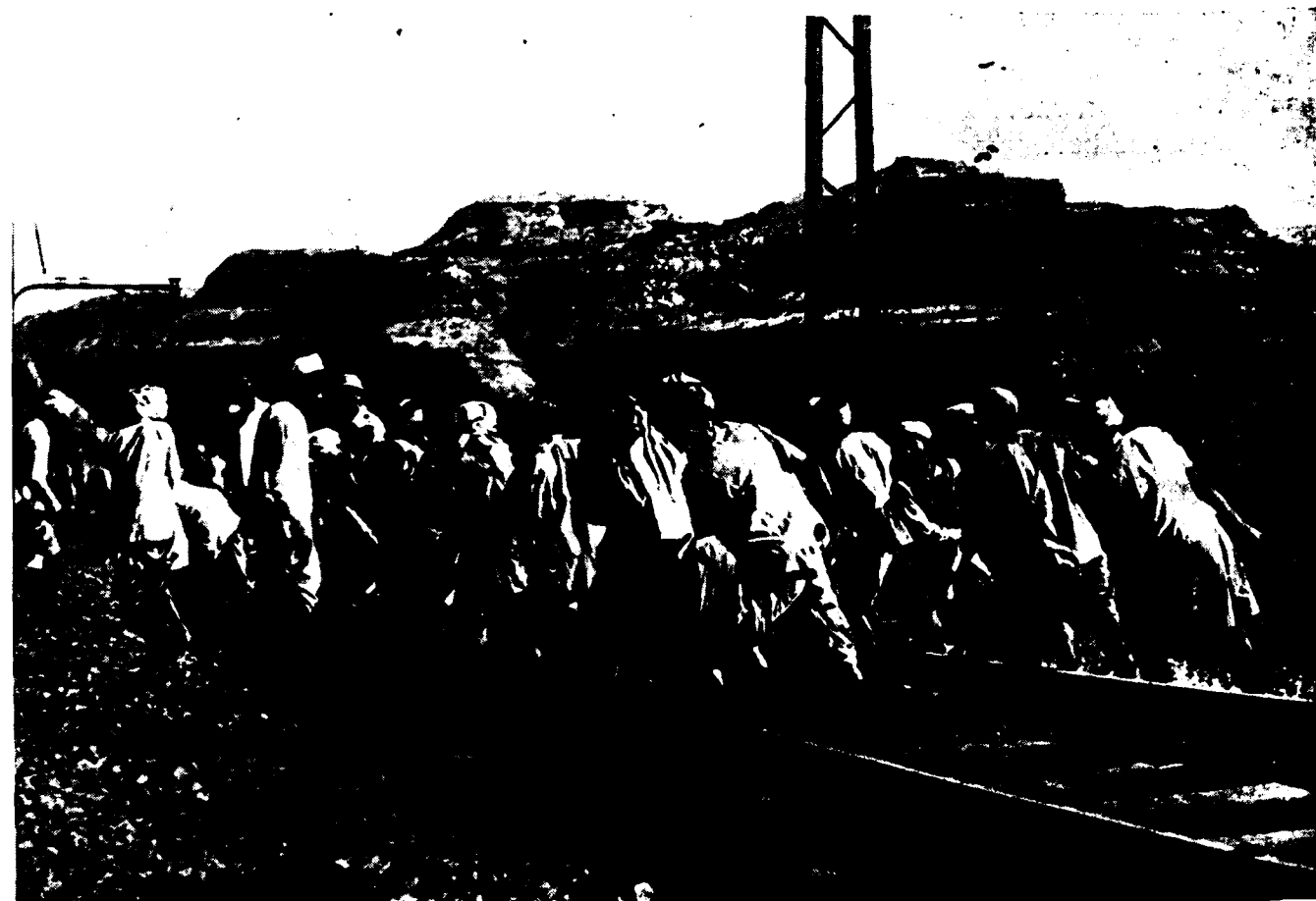
Indian gangmen engaged in operation of track slewing.
