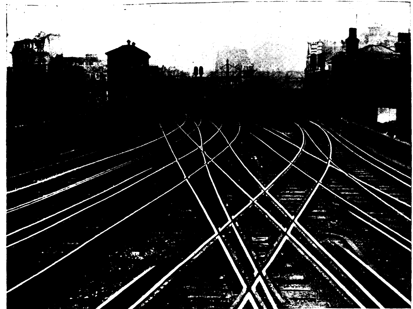
Borough Market Junction—Rolled Manganese Steel Crossings before renewal. (British Railways)
