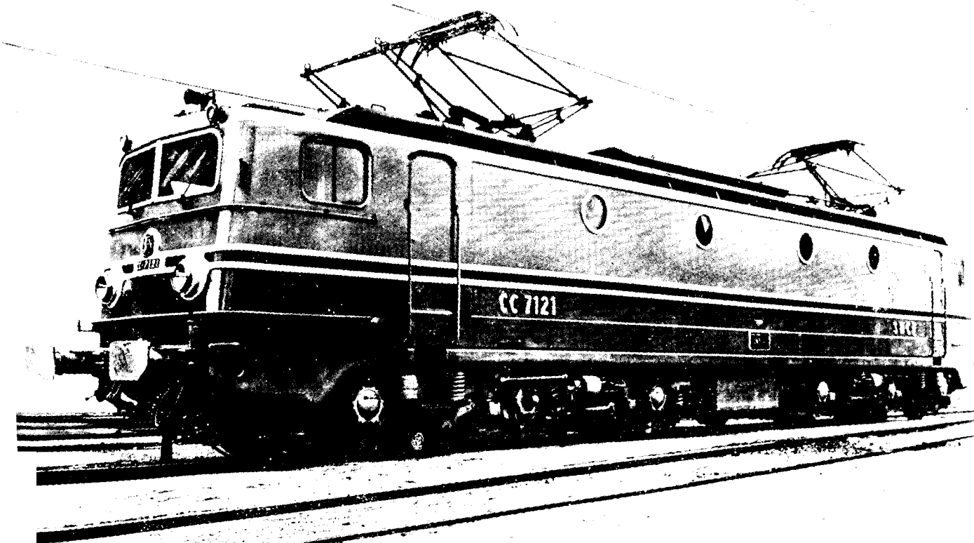
ALSTHOM Electric Locomotive CC-7121 of the French National Railways, which beat the world record at 152 miles/hour on 21/2/54.
