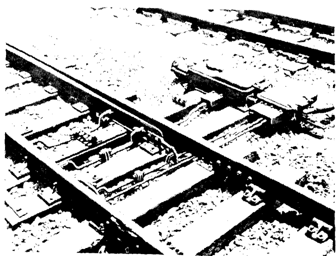
Type HB Combined Point Machine at Krugersdorp, South African Railways.
