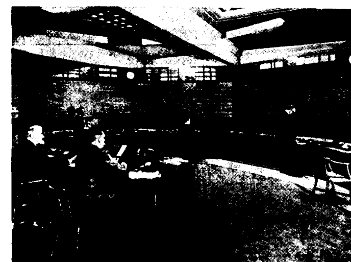
Interior of York Signal Box showing illuminated diagram and console of one control route switches.
