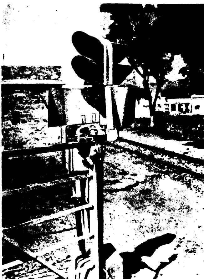
Two aspect electric gate lamps worked by contacts on gates.
