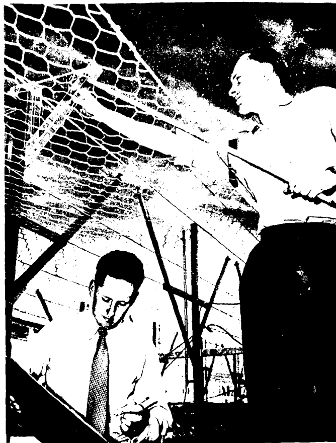
5. Detail of a new type of 'radio telescope' during installation at St Mary's, 30 miles from Sydney, New South Wales, for the Commonwealth Scientific and Industrial Research Organization. Two long thin arrays are arranged in the form of a cross (N-S and E-W). Either array separately has a fan-shaped beam of reception; from the two together an effectively pencil beam is obtained ( \frac{1}{4} beam width). The arrangement was designed by Mr B. Y. Mills.
