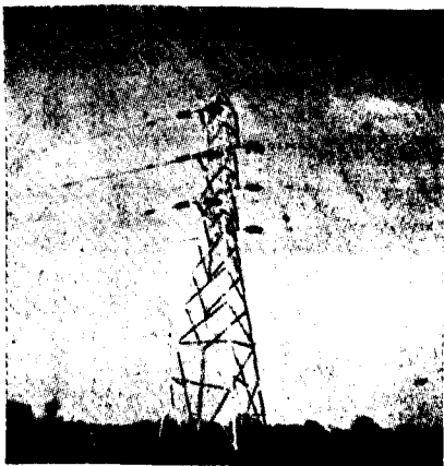
Figure No. 2. A 66-kV double circuit transmission line strung with ACSR "DOG" 16×.186" aluminium/7×.062" steel.
