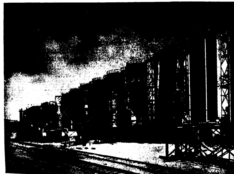
Plant for Production of 50% Nitric Acid.
