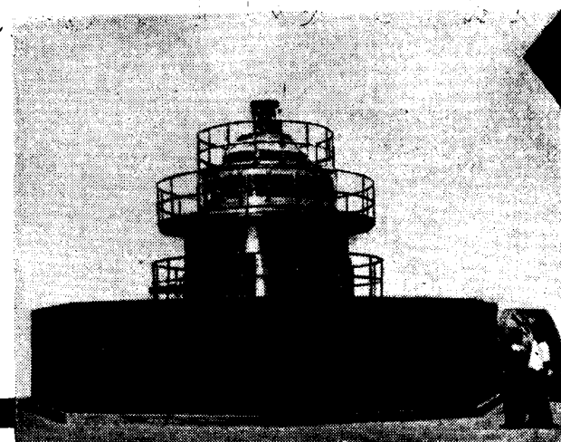
'English Electric' 38,000 KVA Transformers installed at the Delhi Grid Sub-station distributing BHAKRA NANGAL POWER to Delhi.
