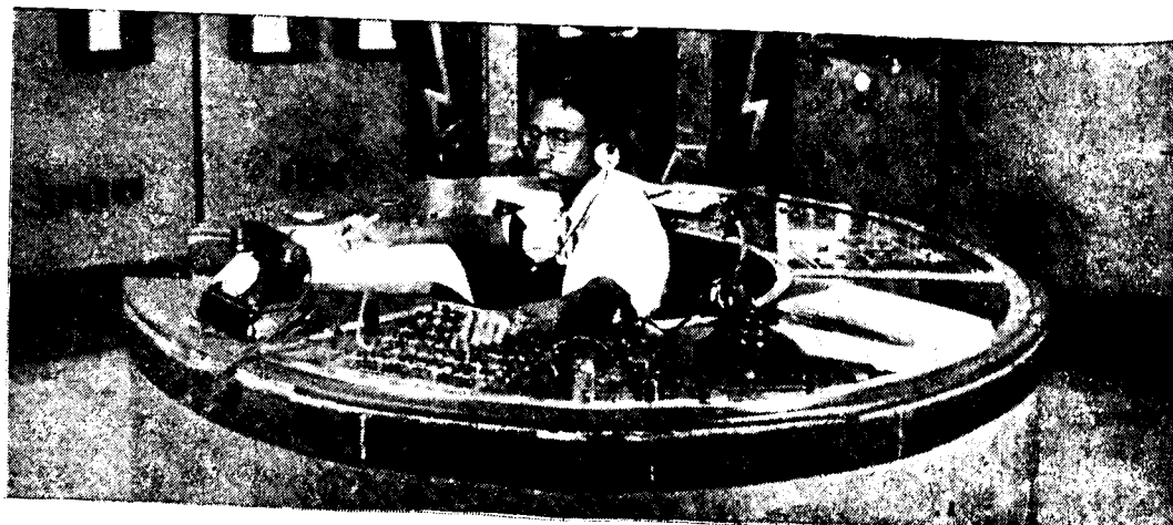
A Section Controller at work
