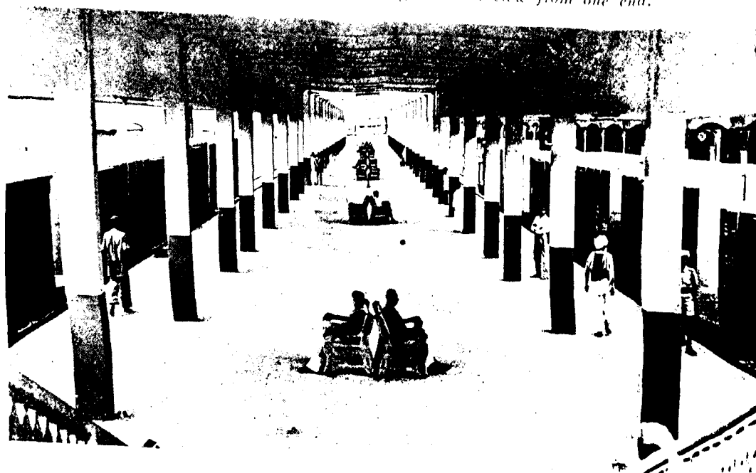
Reinforced cement concrete covering - interior view from one end.
