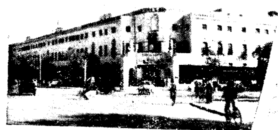
SCINDIA HOUSE, NEW DELHI Electrical Contractors S. K. Singh & Company, New Delhi Architects Walter George, Esq., A.R.C.A. (London), F.R.I.B.A.
