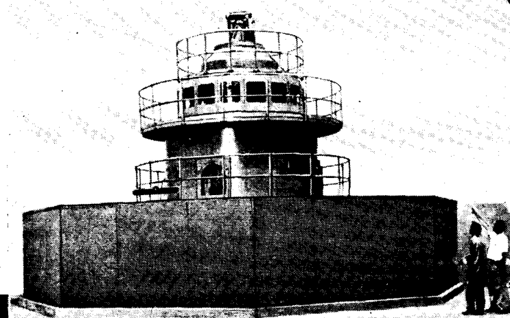
'English Electric' 38,000 KVA Transformers installed at the Delhi Grid Sub-station distributing BHAKRA NANGAL POWER to Delhi.
