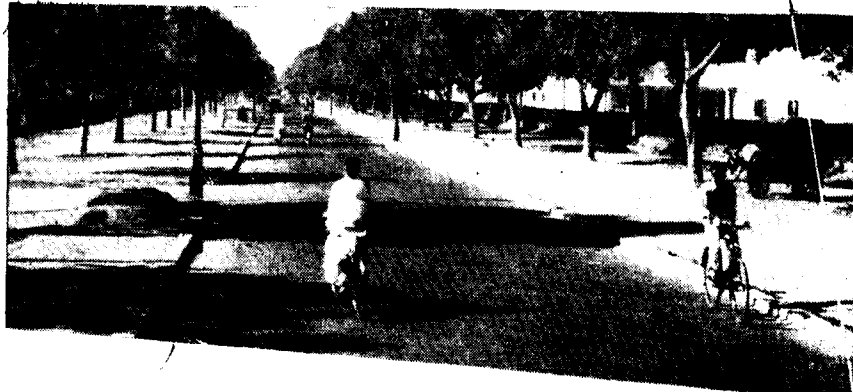
Ferozeshah Road —Surface painting with Mexphalte 80/100 originally and repainted with Mexphalte 80/100 during 1945/46.
