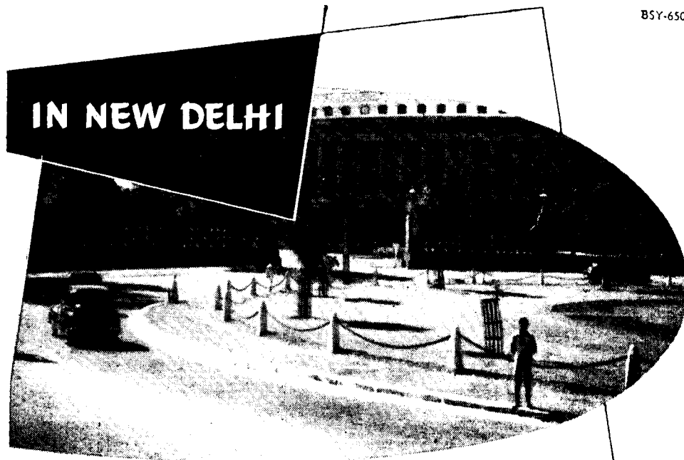
Traffic Rotary at Council Chamber —1" Shell-macadam with Mexphalte 80/100 (fluxed with K) laid during October 1952. Subgrade is surface dressing on WBM.
