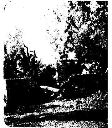
Cyclone Damage in Tiruch
