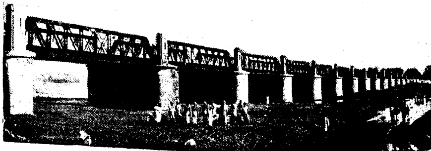
Caleroon Road Bridge, Trichinopoly District, 24 spans of 100-feet on Masonry Piers.
