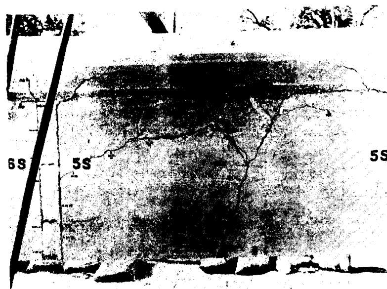
Photo 4: View showing the Cracks at the Centre of the Beam on the South side.
