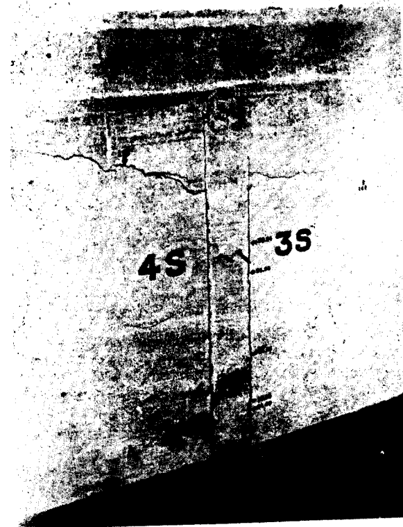
Photo 6: Another View Showing Cracks on the South Face of the Beam.
