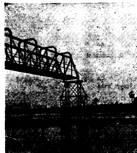
A portion of the Screw-pile bridge
