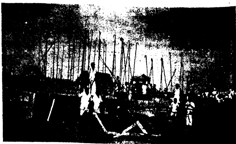
Start of Well Construction
