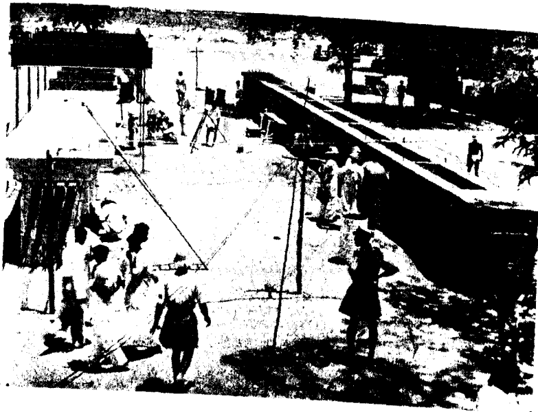
Photo 2: Test beam under load. Beam on the right is ready for prestressing.
