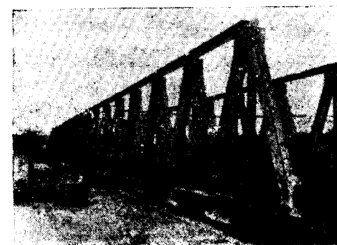
The Raidak Bridge—Callender-Hamilton truss assembled on the bank before launching.
