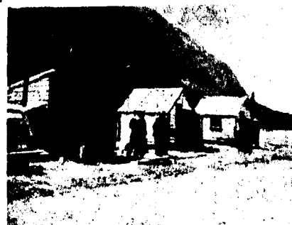
Photo: 16 Temporary work-site quarters
