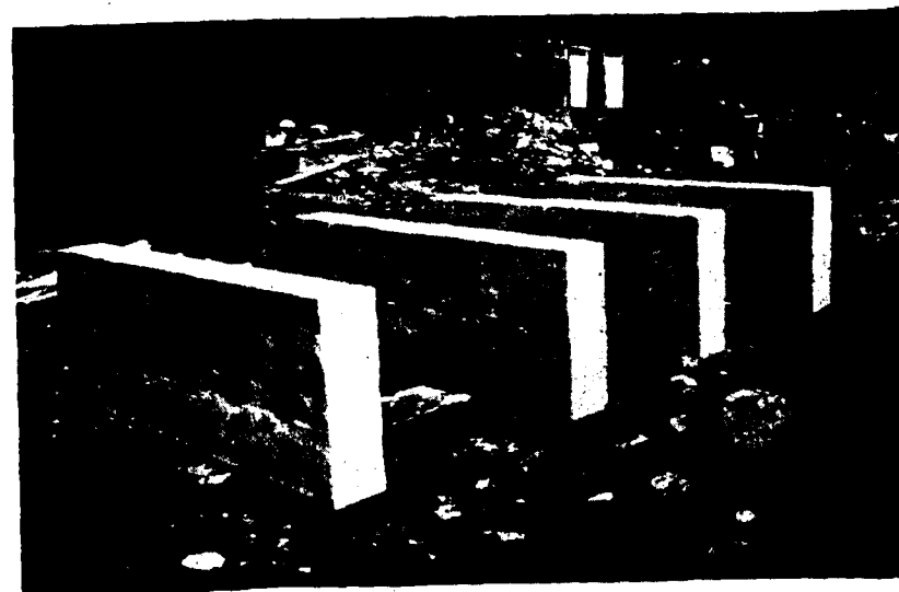
Photo 1. Abercrave Bridge—Precast Anchor blocks
