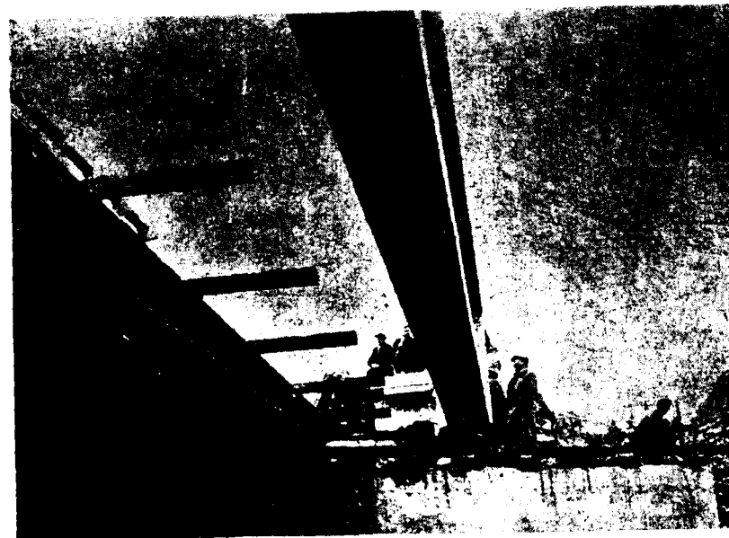
Photo. 6: Abercrave Bridge—Precast girder placed on bogies, being moved sideways.
