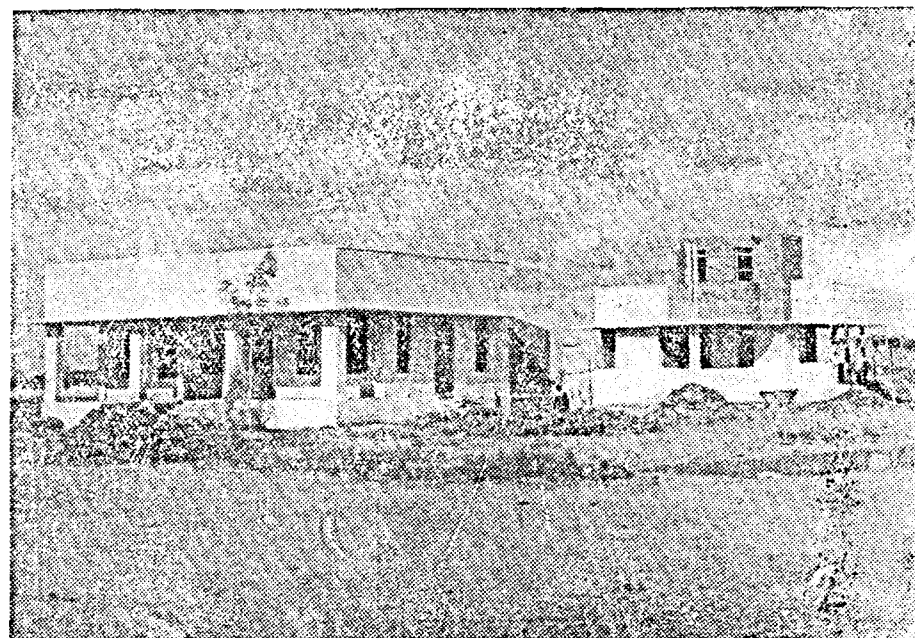
Two typical houses built by the Babujinagar Rural Housing Society at Amaravathi, Guntur District.
