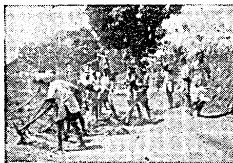
COMMUNITY PROJECT: Villagers at work on the Yekkar-Niddodi Road in the South Kanara Community Project Area.
