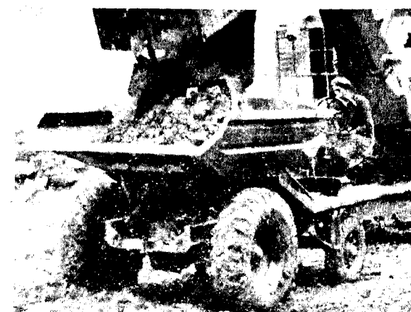
AVELING-BARFORD SHUTTLE DUMPER 4½ c. yard capacity
