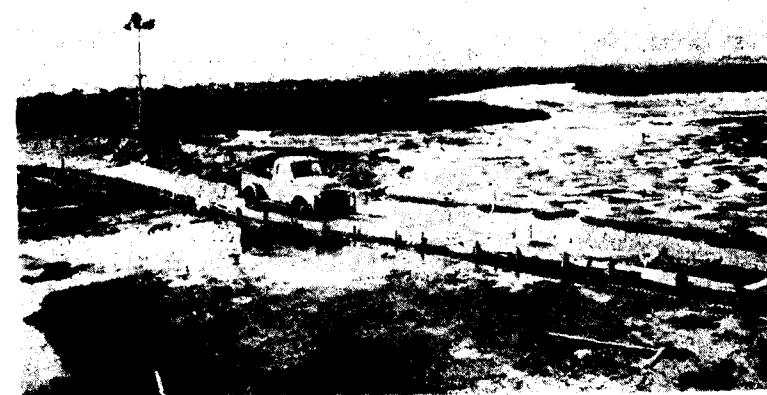
Roadway poured partway across tidal flat at Point Mugu, Calif.
