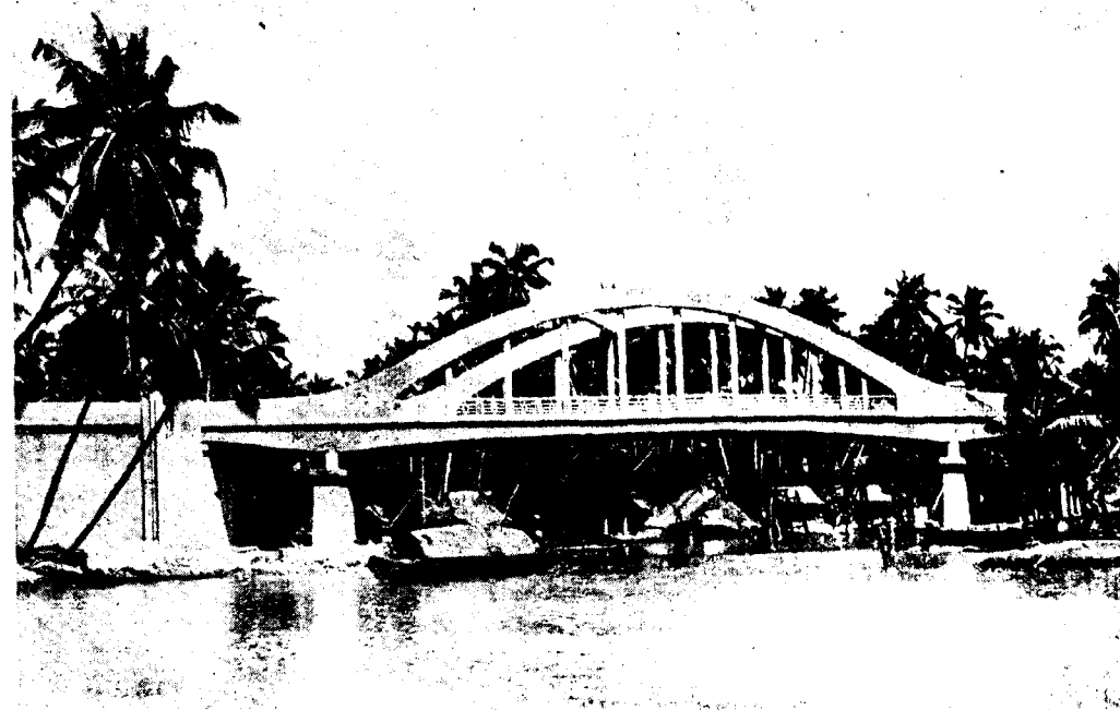
Another view of the completed bridge. (The old bridge is seen in the background)
