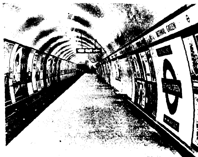
Modern Tube Railway Station on London Transport Lines
