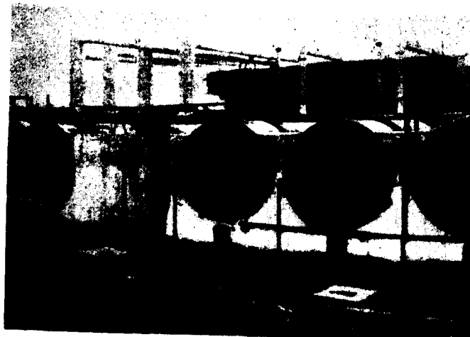
3. Distillation: a bench of stills used early in the present century for the distillation of petroleum. Each still held some thousands of gallons. The earliest continuously operating plant was evolved from stills of this type.
