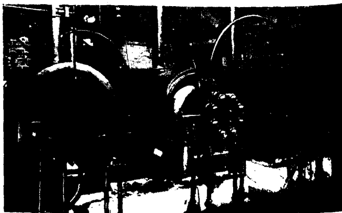
8. Hydrogenation of coal: replica, erected at the Fuel Research Station, Greenwich, in the late 1920s, of the original pilot-plant (at Mannheim) for the Bergius process. ( Fuel Research Station, Crown copyright. )
