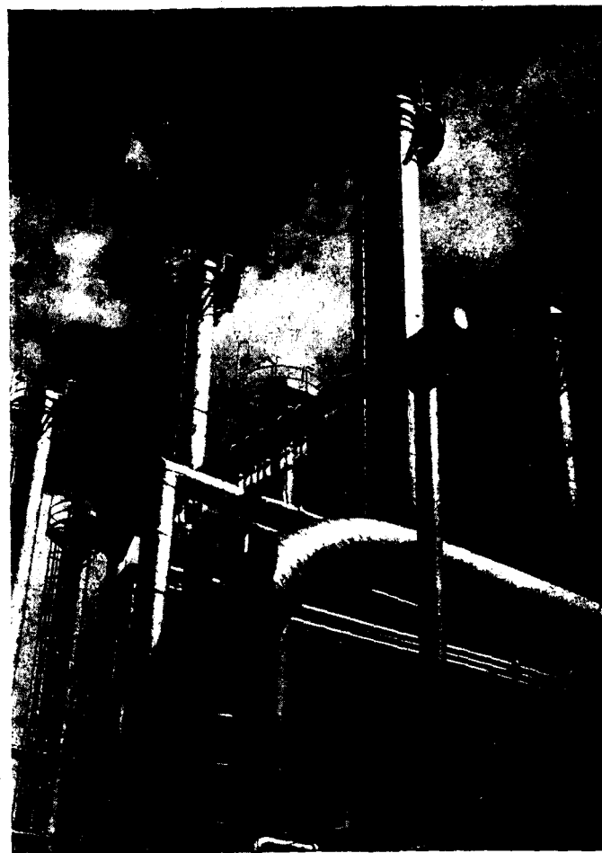
1. Distillation: fractionating towers on the distillation unit, Shell chemical plant, Stanlow (by courtesy of the Shell Petroleum Company, Ltd). The evolution from laboratory-type equipment to continuous, large-scale operation is shown in the three following pictures.
