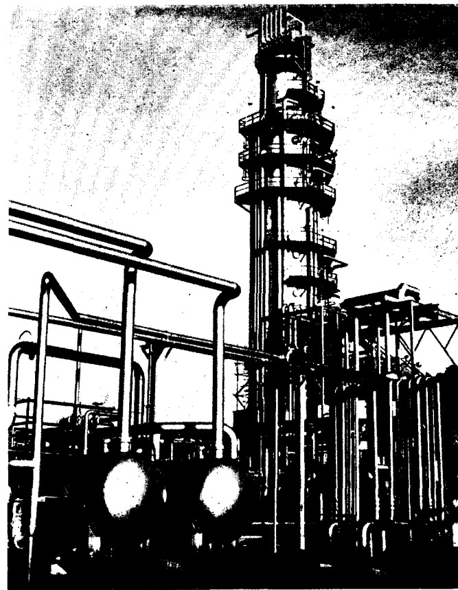
4. Distillation: continuous operation. Fractionating tower of single-stage unit for the fractional distillation of crude petroleum at the Esso refinery, Fawley. (By courtesy of the Esso Petroleum Company, Ltd.)
