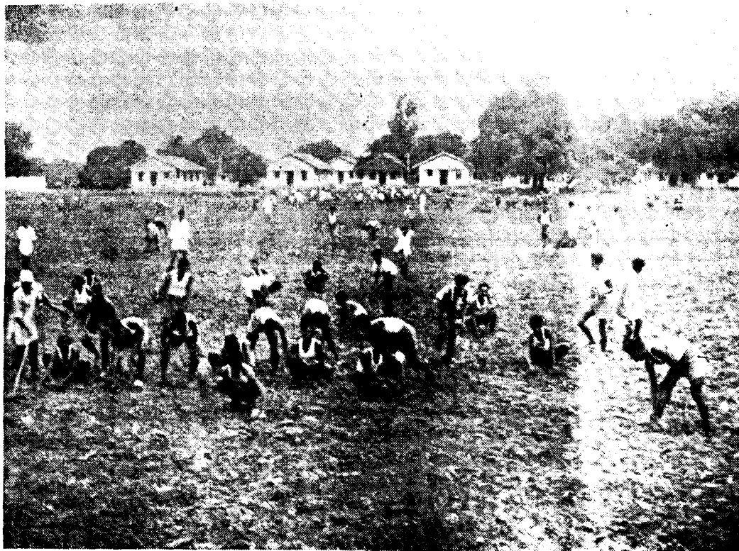
Students at work preparing a New Sports Field at the College
