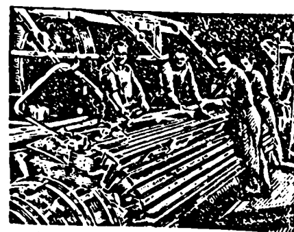
Assembling copper coils in generator field rotor.
