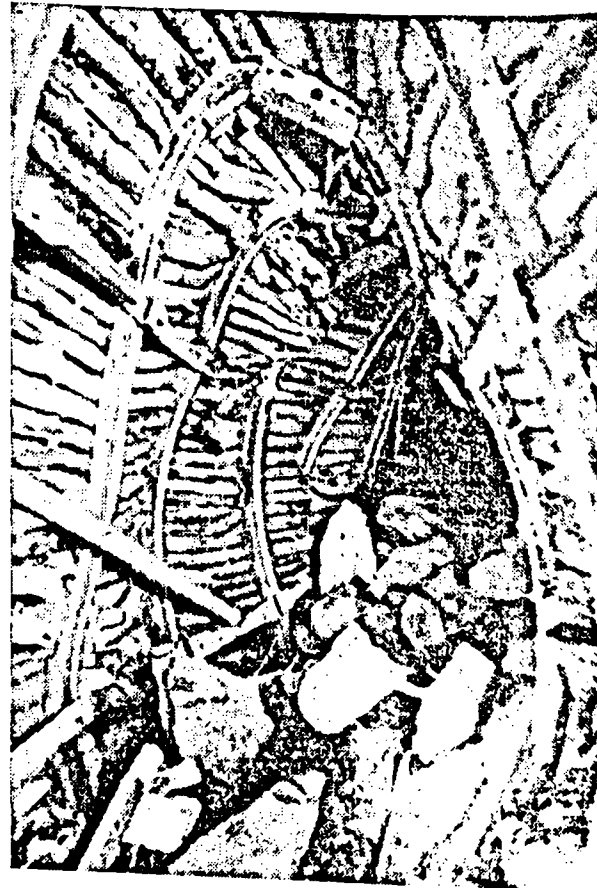
Steel setted level after a rockburst.
