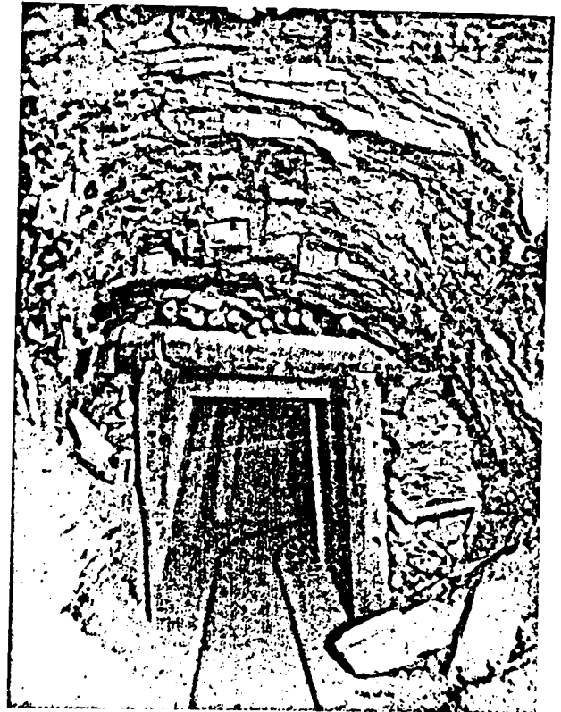
Timber setts in a level.
