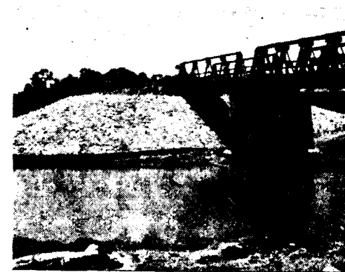
Gadadhar Bridge East Abutment—showing scour against the toe wall of bank.
