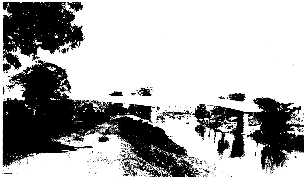
The Taldanga Bridge. The railway bridge upstream can be seen in the background.
