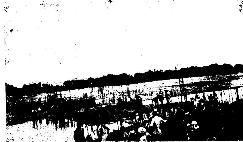
A view showing the bridge under construction.
