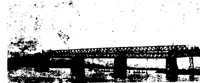
Photo No. 7—Special centering leaves the river unobstructed and work can go on in all seasons.
