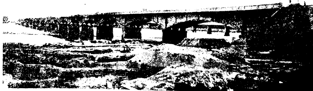
The Kathjuri Bridge.
