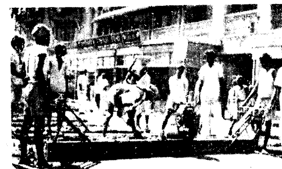
C. H. Johnson self-propelled screed vibrator.
