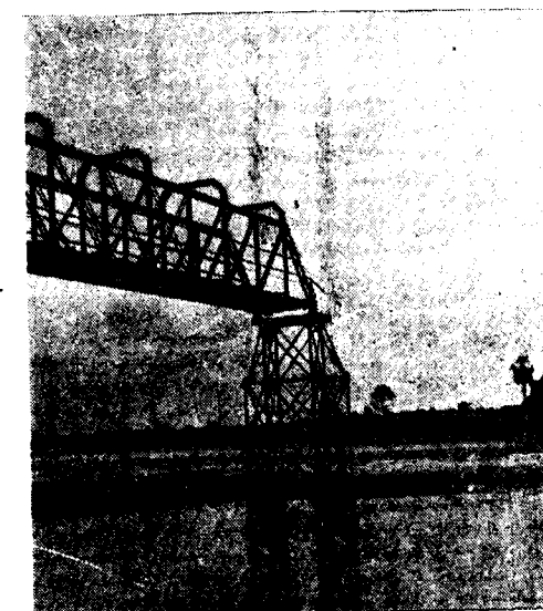
A portion of the Screw-pile bridge
