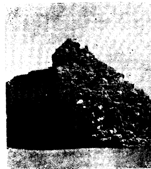
Remains of a collapsed abutment.
