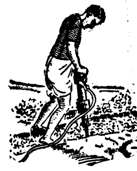
PAVEMENT BREAKING
