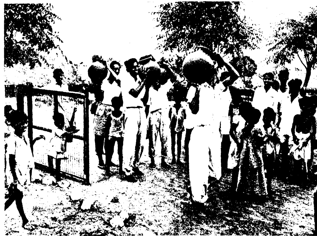
CARRYING WATER FOR THE BUILDING FROM THE WELL
