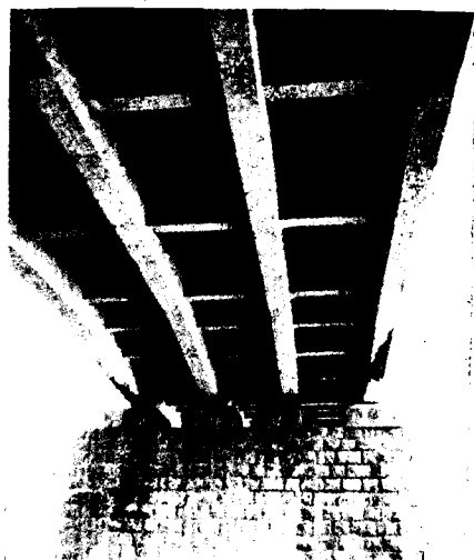
Photograph No. 3. A view from below showing the T-beams and cross beams.
