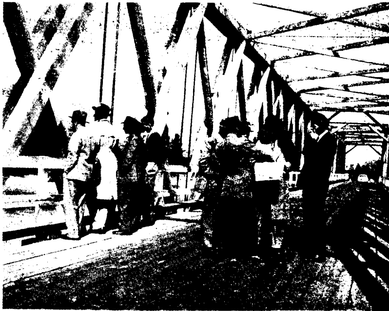
Photograph No. 2 (above) and 3 (below): Two views of the timber Howe Truss Bridge, over the Columbia River, near Canal Flats, British Columbia, (Para. 12.2.)
