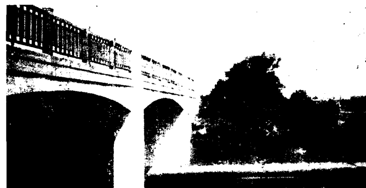
Photograph No. 6 A Grade Separation on the Elizabeth Regina Highway. (R. C. Rigid Frame Structure) (Para. 14. 3.)
