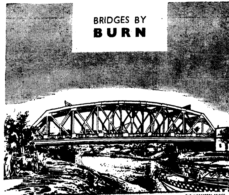
THE KIDDERPORE BRIDGE
