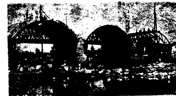
View showing the work in Progress.
