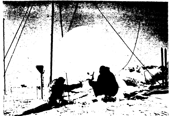
7. Meteorologists prepare to launch radiosonde-rawin balloon from Maudheim. Launching in a gale, with surface-blown snow, needed all hands.
